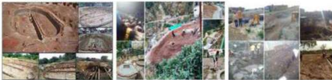
Under Construction Fixed Dome Bio-Gas Plants (Totally Underground)
