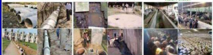
Sewer Line Laying (Big Dia) Problems
