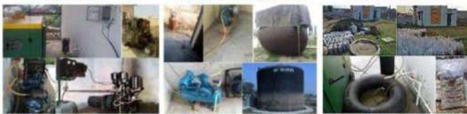
Electricity Generation From Bio-Gas
